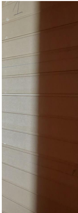
Photo 2 Close-up of the vertical outer edge of the long wing at a height of 500 mm above the floor of the trolley
